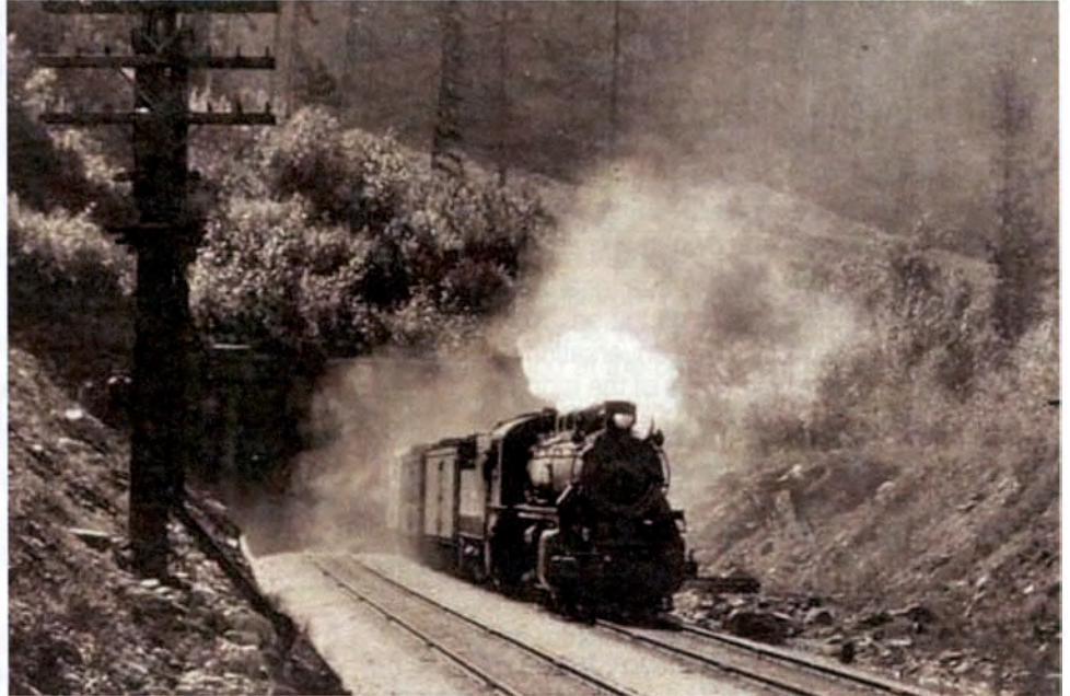
A CPR eastbound locomotive blasts out of the East Portal of the Connaught Tunnel on double track which dates this photo prior to 1959 as that was when the double track was replaced by single track.
